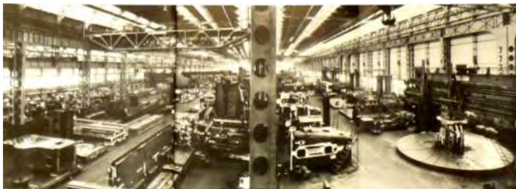
Interior view of the shed Innocenti, steel elements production, '50.
