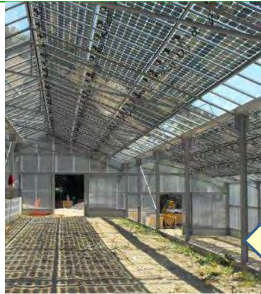
Productive part: PV roof
