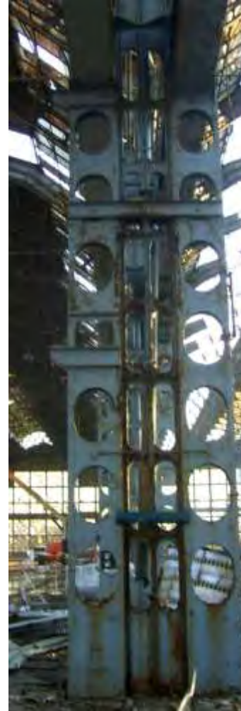
Steel structure of the column.
