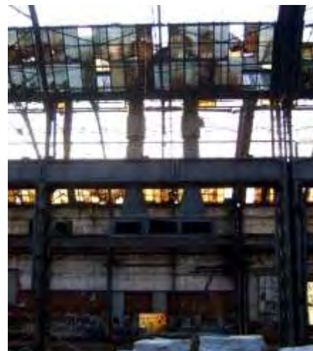
Bridge crane structure
