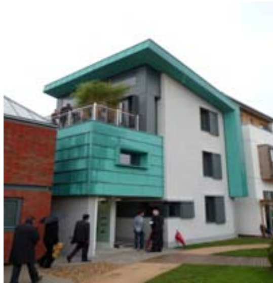
The Greenhouse, Barratt
