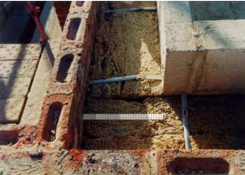
'BedZed': cavity wall, 300mm!!
