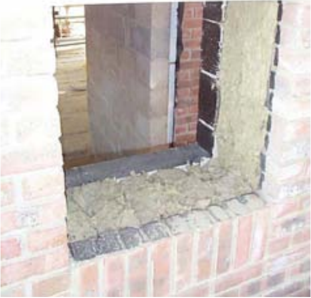
'The Green House': cavity wall, 250mm!!
