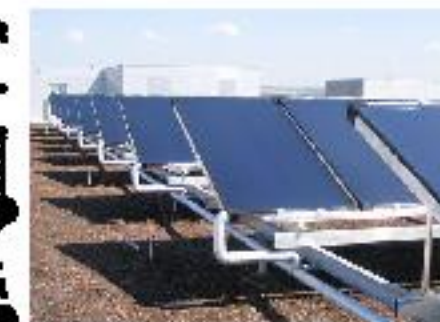
INCLINED PVS ON THE HORIZONTAL ROOF TO ACHIEVE MAXIMUM SUNLIGHT CAPTURE
