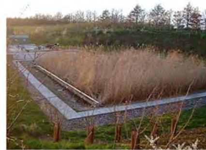
reed bed sewage treatment systems (biological filtration-aerobic bacteria)
