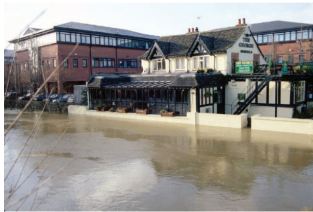
2 Flood in Oxford, UK, Dec. 2008, one of several floods during that winter and thereafter. Building on floodplains has been a widespread unsustainable practice in many countries. In recent years this has caused repetitious flooding of residential and other areas, affecting structures and causing health problems due to humidity and mould growth. (Photo: I.A. Meir)
