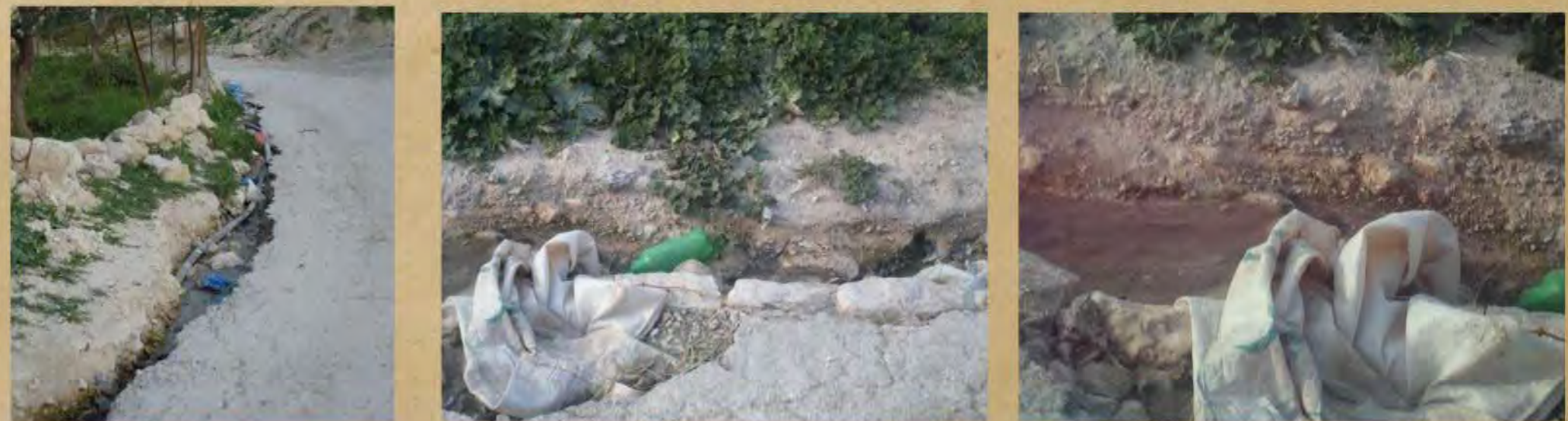
Existing situation with the open sewer in the street
